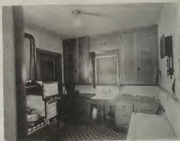
FINE EXAMPLE OF BUILT-IN CUPBOARD, CABINET AND SINK. THE TWO OPEN SHELVES AT EITHER SIDE OF SINK SERVE AS WORK TABLES, DRAINBOARD AND GENERAL UTILITY WHERE SPACE IS SMALL. DISH PAN, DRYING PAN AND WASTE BASKET WELL LOCATED UNDER SINK. WINDOW ABOVE
